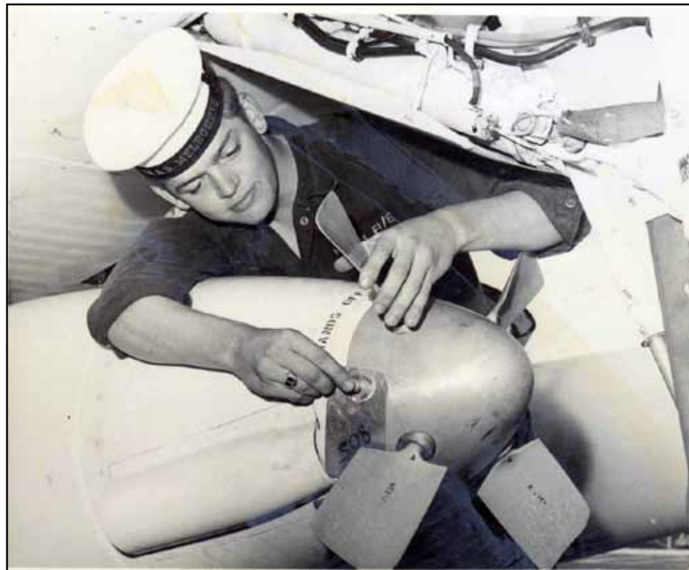
Navy PR photo (hence cap on flight deck). Dutchy secures an A-4 tanker buddy store turbine, April 1969, South China Sea. Photo via author.
