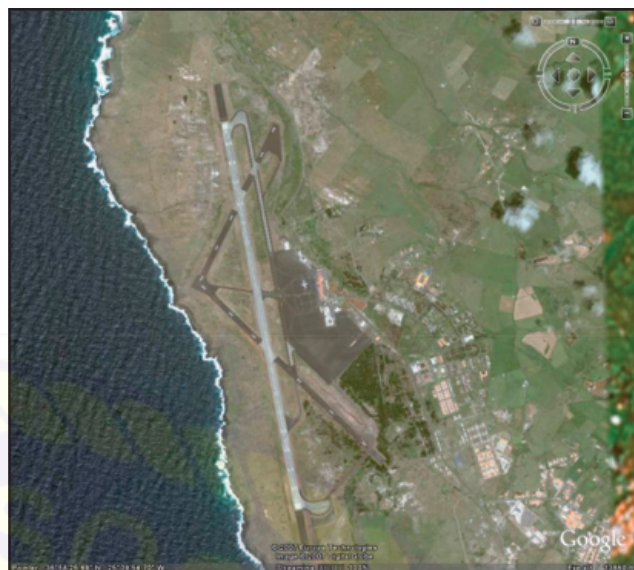
Aerial view of the airfield at Santa Maria Island, scene of the VMA-223 accident during the strenuous 1986 TRANS-LANT.
